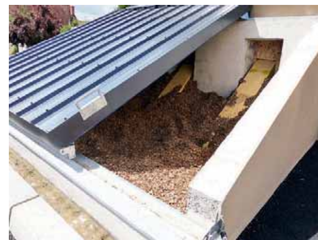
Chaufferie bois EIAT Château-Chinon
